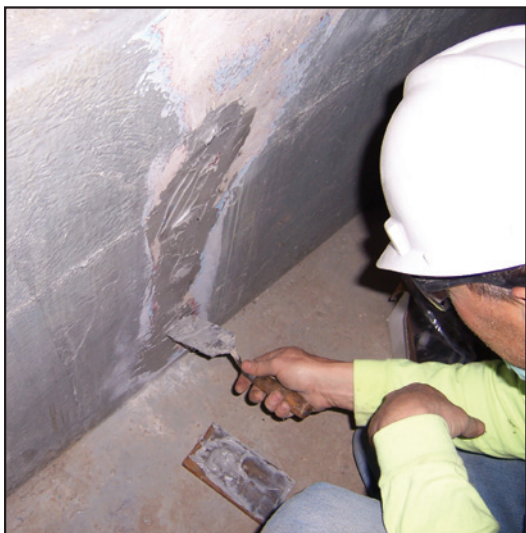
Treating crack with ChemLine ® Caulk.
