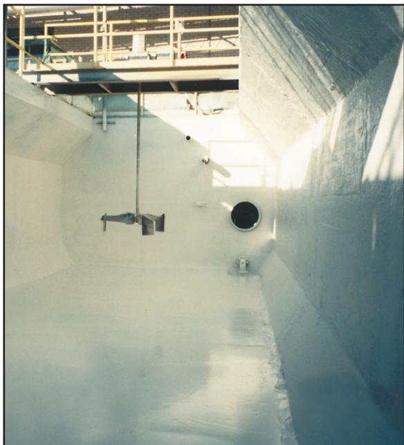
Finished ChemLine® Primer application over concrete surface.
