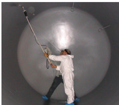
Tank interior coated with ChemLine®
